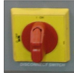
Figure 3. Disconnect Switch.
